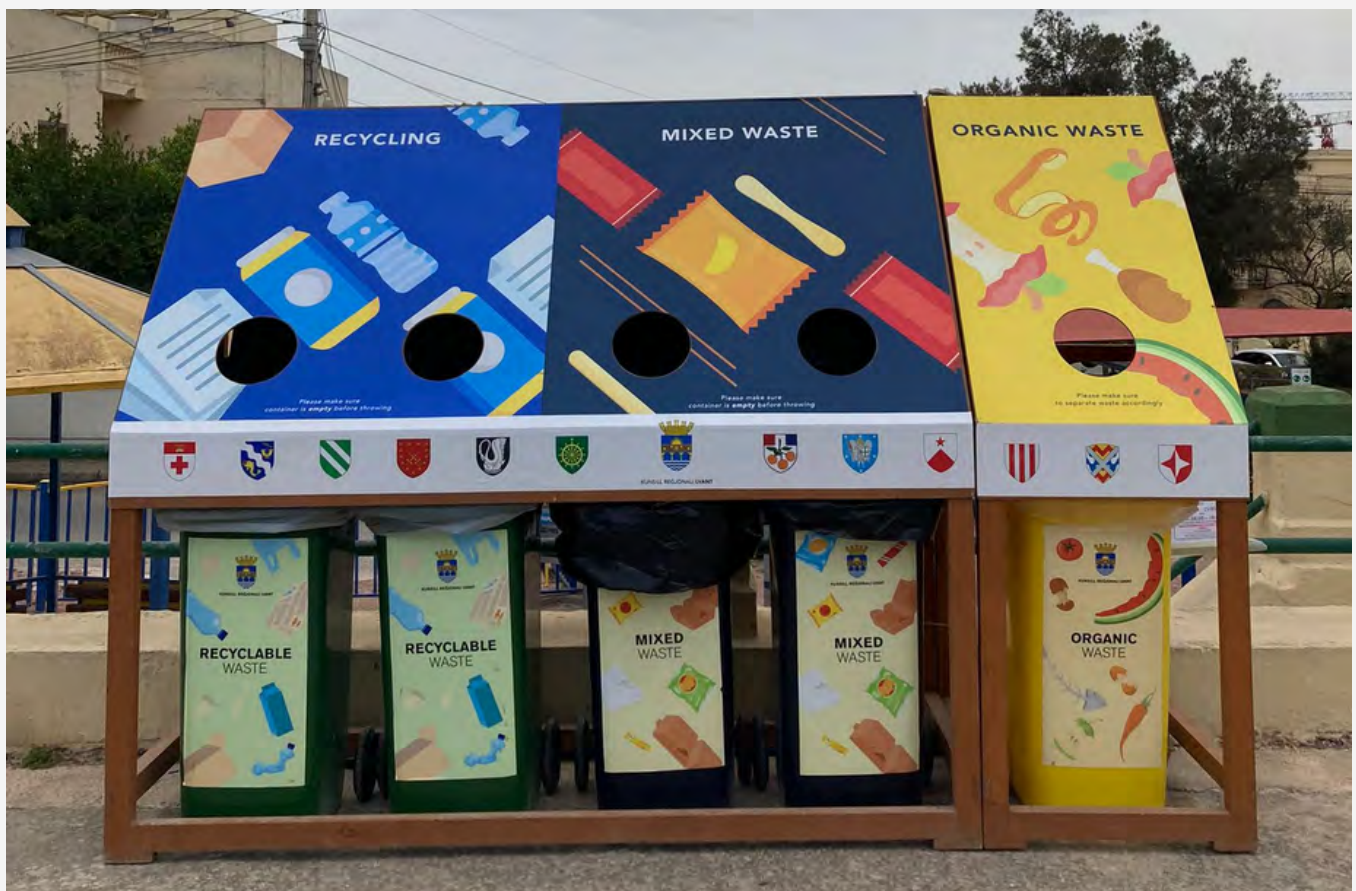
Bin Structure installed at Iklin for Festa Fjuri
